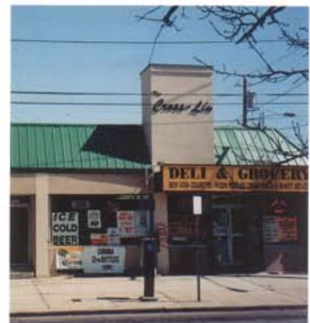
Storefront fascia and mansard panels fabricated from supplied drawing.
